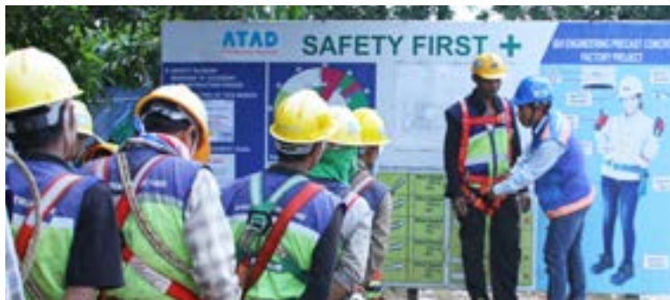
Safety sign always shows during work in progress
